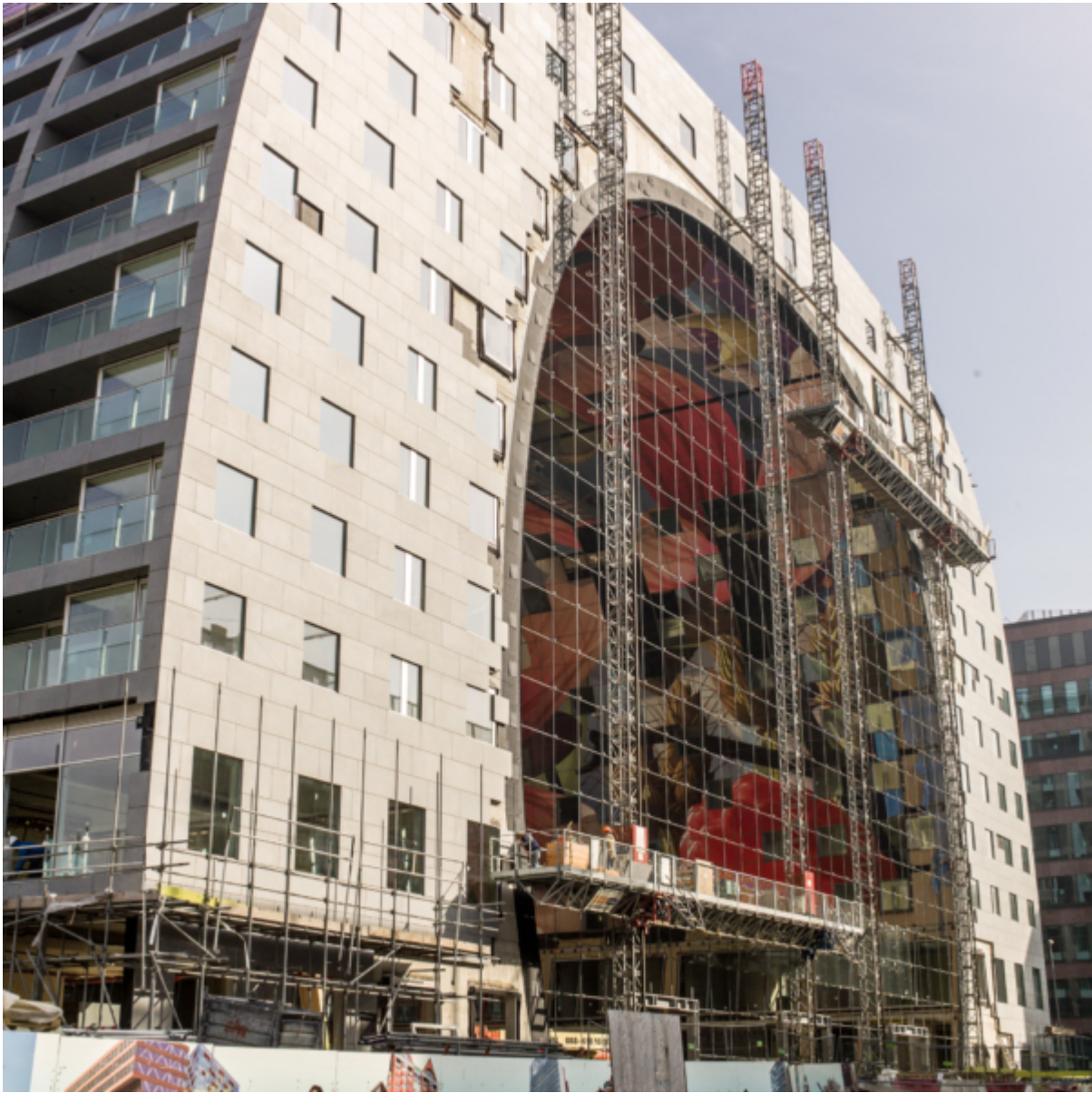
Building the new Market Hall
